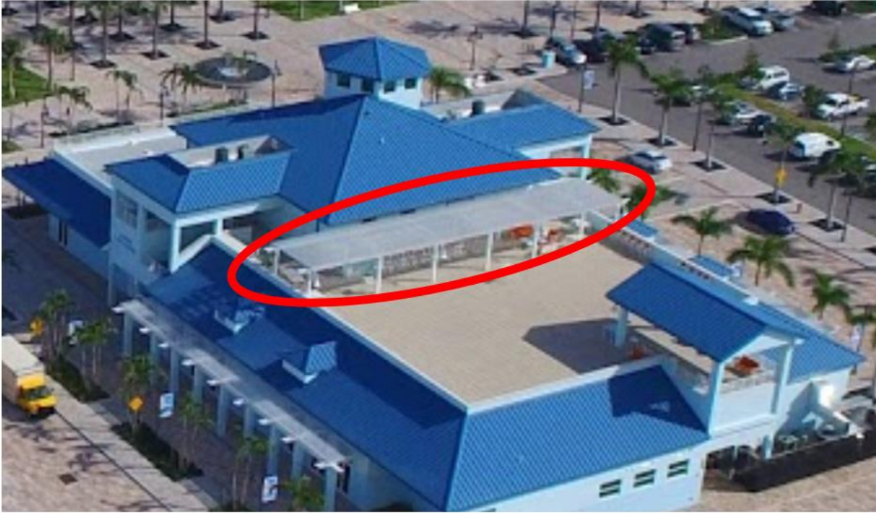
Proposed Installation Area
