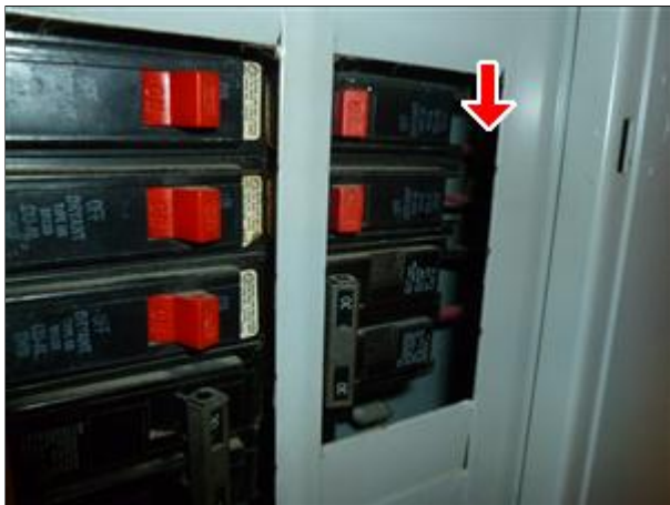
Exposed Panel - Suite 3
