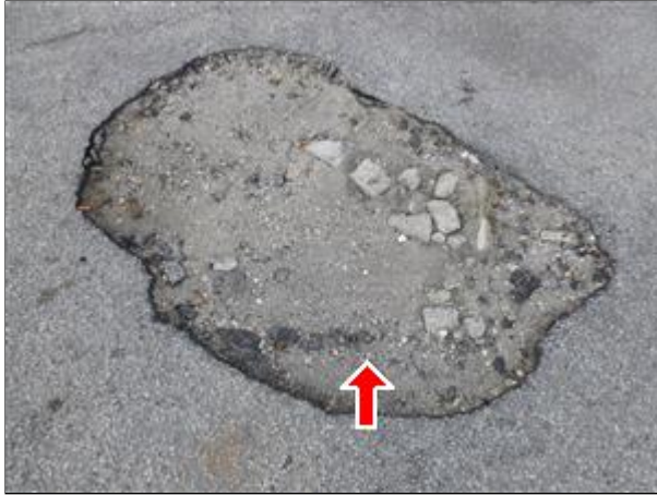
Damaged Asphalt
